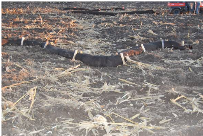
Figure 1. Filter socks in position. RTV used for transport in background.
